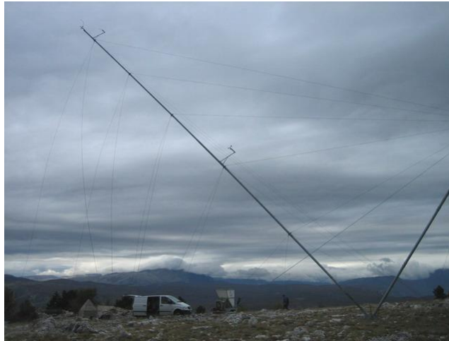
Fig. 4 Podvelez /MaliGrad - Lifting 30 mast
