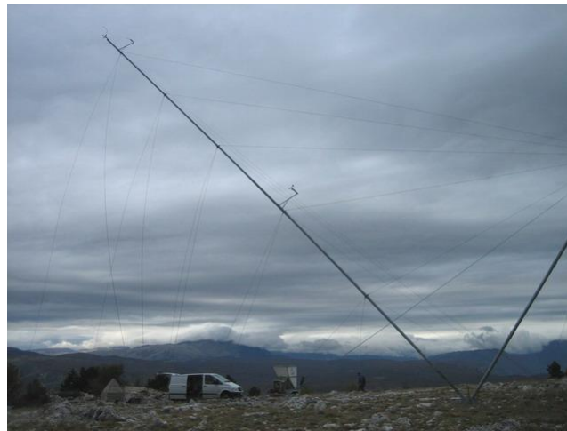
Fig. 4 Podvelez /MaliGrad - Lifting 30 mast
