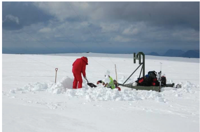
Figure 4-5: Accessing power system in a remote location. The whole 2.5-meter high container apart from the air inlet to the engine has been buried. Photo credit: Lars Tallhaug, Norway
