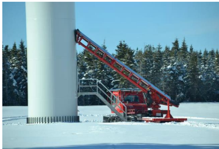
Figure 21: Mobile roof built by GDF Suez at Caribou wind parc to access wind turbines requiring maintenance when there is a risk of ice throw [233]
