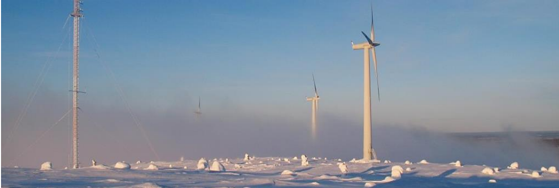
Figure 13: Olos fjell wind farm in Northern Finland (source: VTT)
